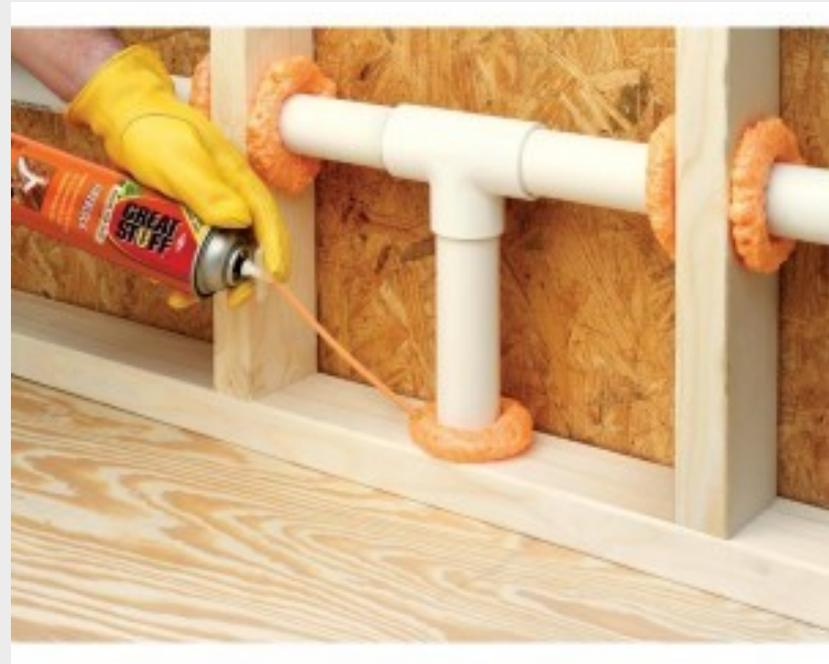
No spray foam products are allowable. Fire-rated caulk may be acceptable, if applied in a workmanlike manner.
