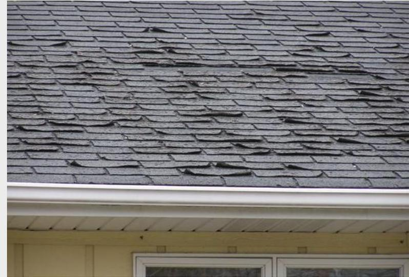
Deteriorated overhang, loose or missing roof shingles, roof flashing and vents shall be repaired/replaced. Roofs leaking badly will require a full replacement.
