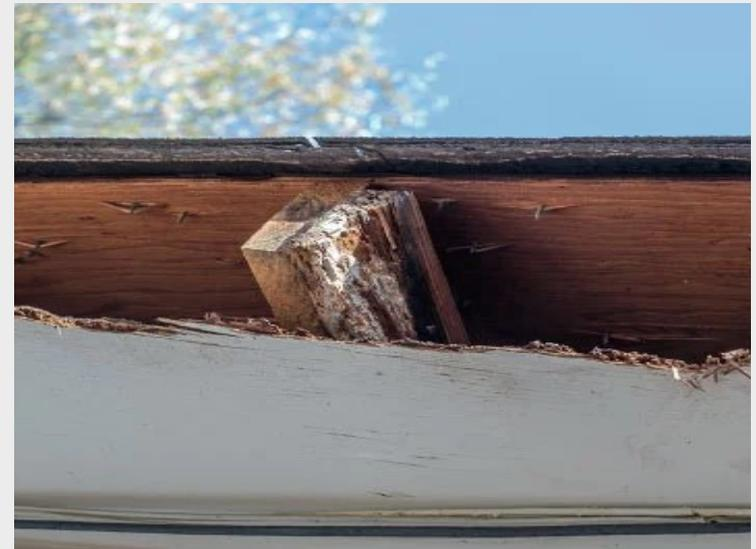
Examples of a deteriorated fascia and soffit that require repair and anchorage to maintain a safe condition.
