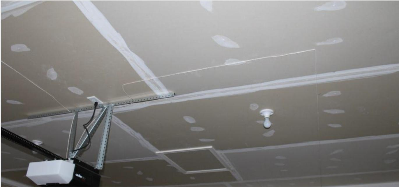
Any openings, in the fire separation wall between the garage and living space, or at pipe and wire penetrations through the floor or wall, shall be blocked. Fire stops may be 5/8" Fire drywall. All drywall joints must be taped with at least one coat, at area bordering living space. A rated door of 20 minutes protecting the door openings
