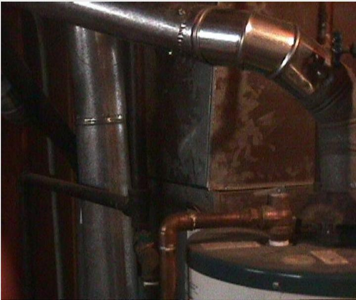
No bright (flimsy) aluminum vent; must be dull (sturdy) galvanized venting.
