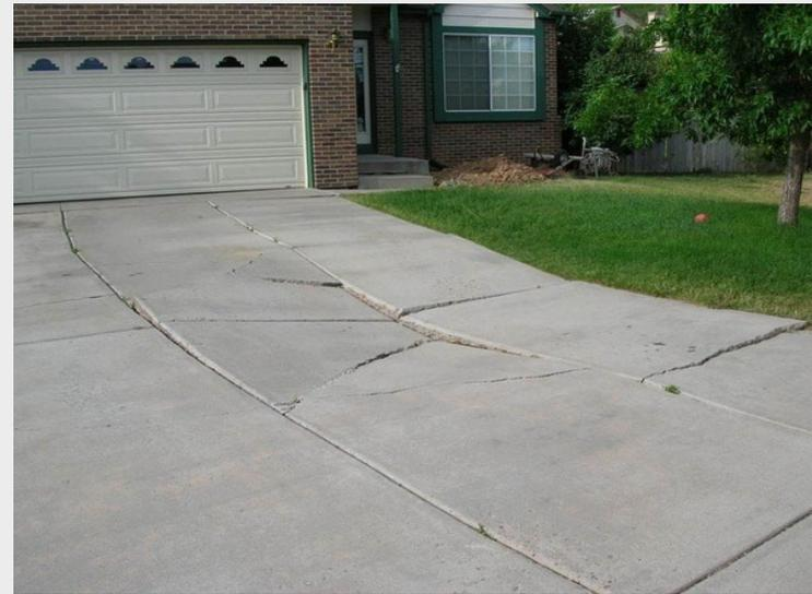
Surface differentials of  $\frac{3}{4}$ " or more on driveways and walkways are a trip hazard and must be leveled.  $\frac{3}{4}$ " cracks must be repaired. Gravel driveways must come into compliance with city code.
