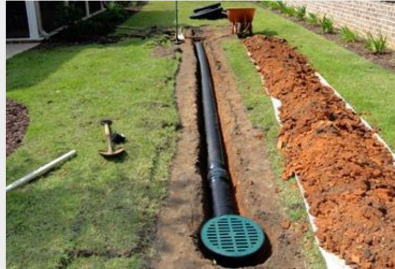
Roof drains, gutters and downspouts shall be maintained in good repair and free from obstructions. Roof water shall not be discharged in a manner that creates a public nuisance. Drainage/Underground drainage must be keep back 15' from the backside of street curb.
