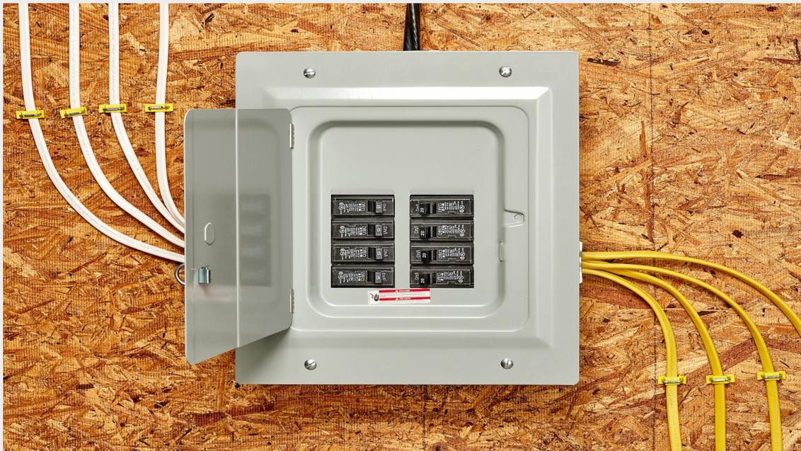
Minimum 60 amp service is allowable. Inspectors check cable clamps and circuits for appropriately rated fuses. Inspector opens box door, but does not remove the box cover to verify circuit installations inside the box.
