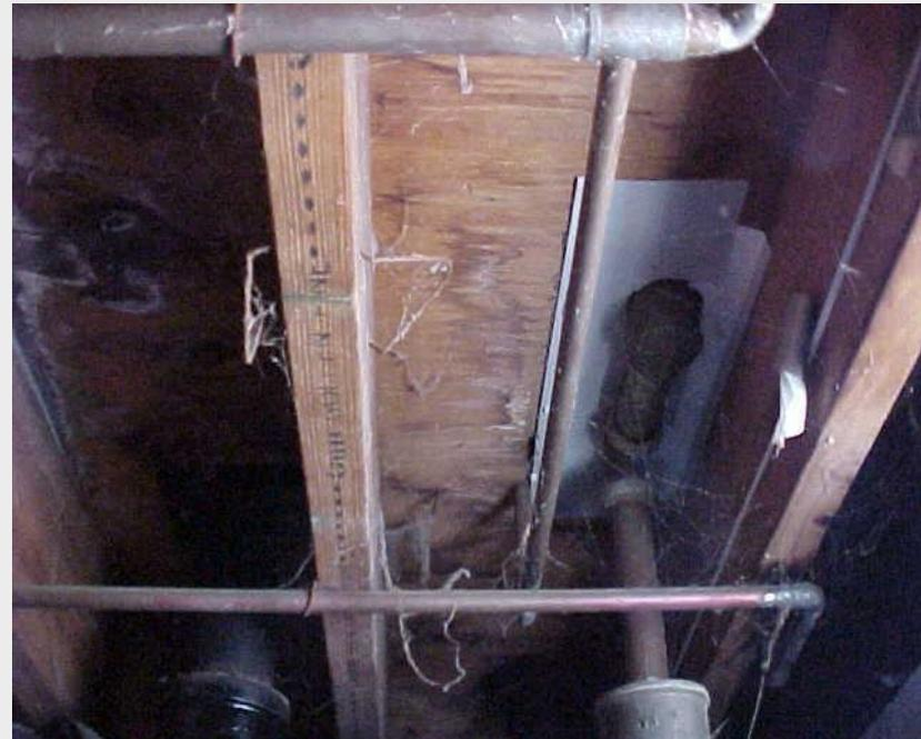
Fire stops at mechanical, electrical and plumbing penetrations must cover any openings; there should be no “daylight” showing where drains and other utilities enter the floor. Fire stop material may include ½ inch drywall, ¾ inch plywood, heavy sheet metal, or approved fireproof caulk.
