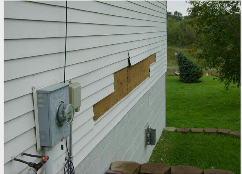
Check for melted, deformed, damaged and missing siding.
