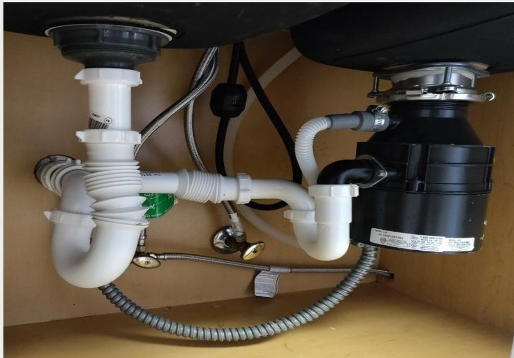
Flex piping on drains is not allowable, per Plumbing requirements. Unvented sinks and vanities will be required to be properly vented by a licensed plumber.
