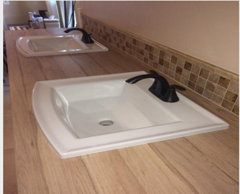
Check for sufficient water pressure, correct hot & cold water connections and leakage around bathtub and fixtures. Caulking at tub surround must be maintained.
